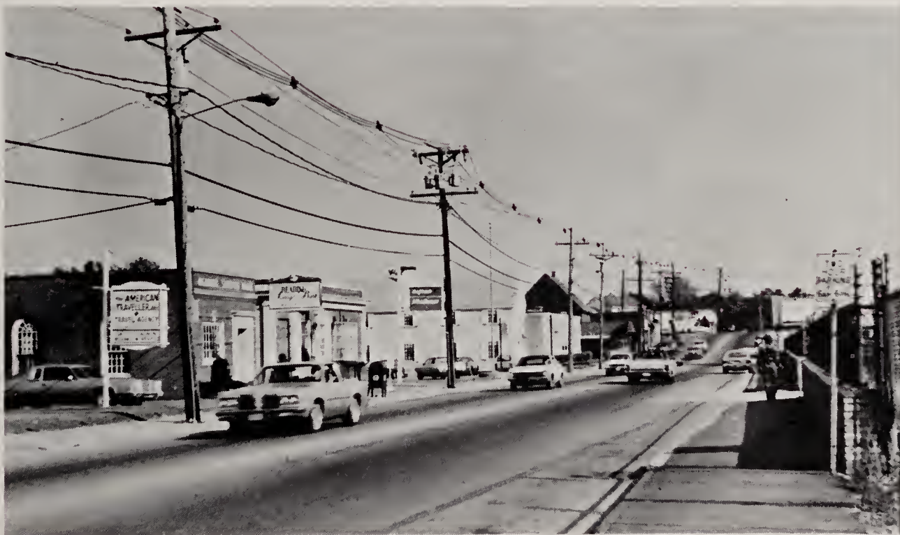
Looking South along Main Street through the "Square" in 1980. Overhead electric and telephone wiring replace the many shade trees.
